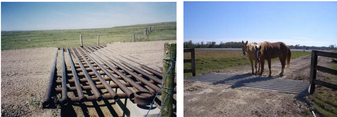
Figure 4. Photographs of Texas Gates
