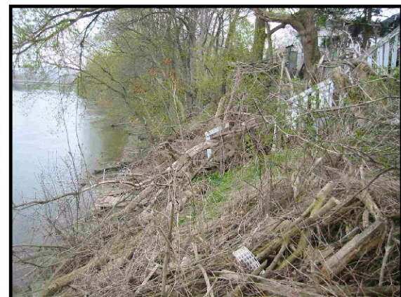
There are many trees along the dyke that are leaning, in addition to dumping.
