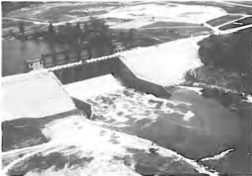
View of Dam and Spillway.
