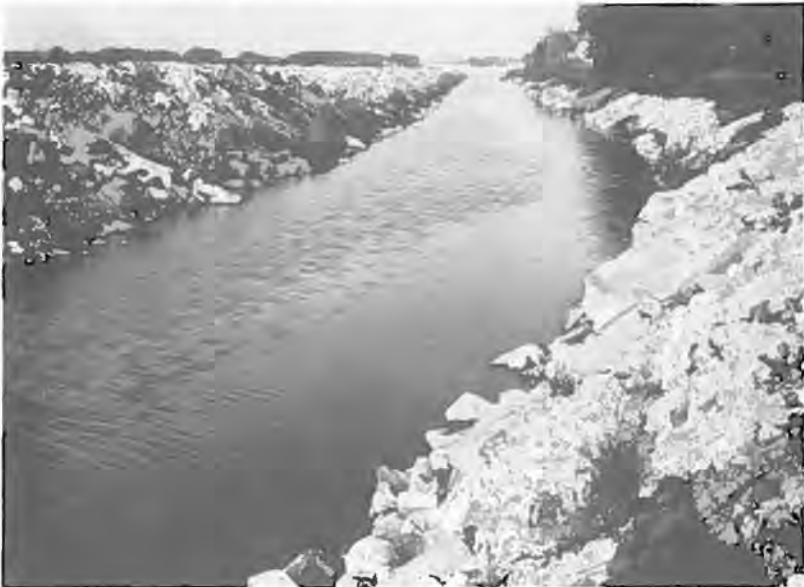
Part of channel improvement between Beachville and Ingersoll.
