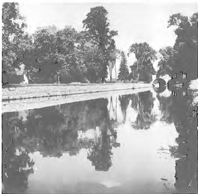
Downstream Channel Improvement, Stratford.
