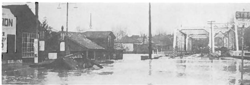
Wellington Street Bridge Looking North.
