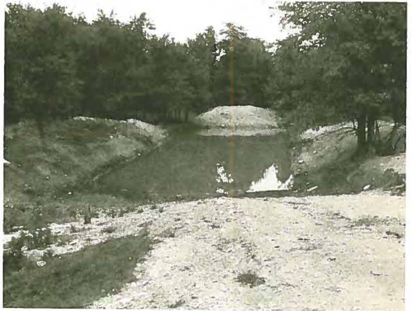
Dug-out ponds like this one near Elginfield are common in areas with ground water near the surface.
