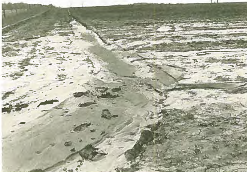
The spring thaw washed out this small gully on a 3 per cent slope near Stratford.
