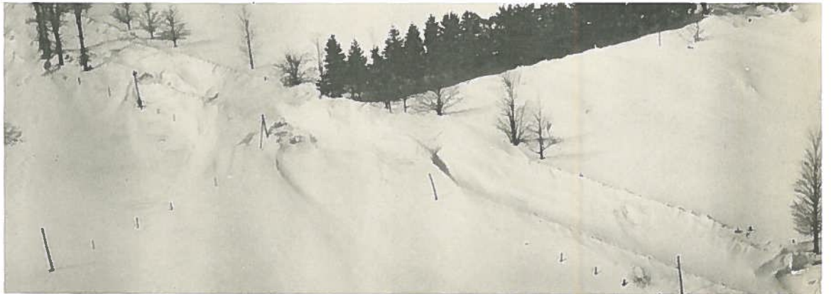
Poorly Placed Windbreak: This windbreak, poorly placed with respect to the highway, has created drifts across the public road.
