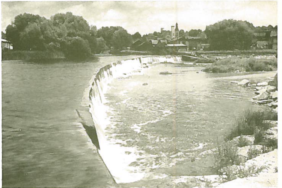
St. Marys Dam—present dam has not sufficient spillway capacity to discharge the high spring flows safely.
