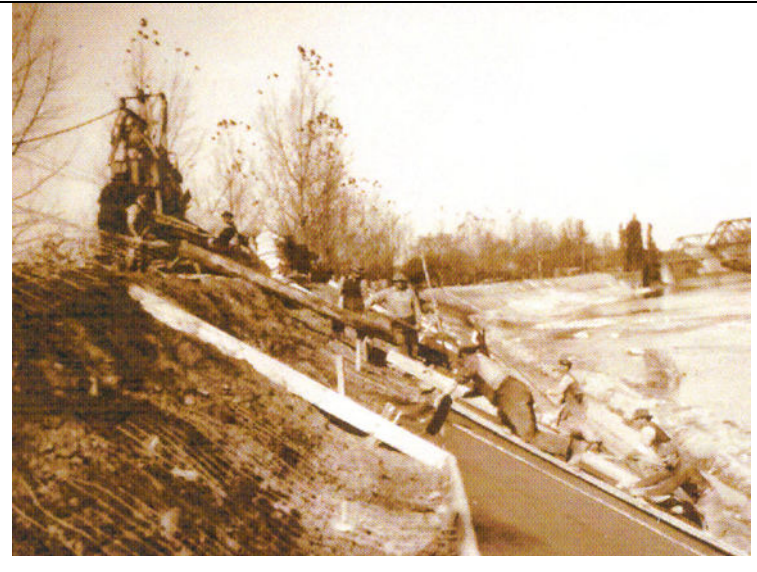
Fig -1 Photo from the 1930's showing the concrete Dyke being formed.
