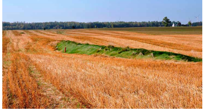
A well built and maintained berm helps control runoff through a natural drainageway on this farm. Thirteen narrow-based tile outlet water & sediment control basins (WASCoBs) and a grassed waterway were installed across this property to control rill erosion.
