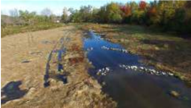
These in-stream rock structures will improve flows and water quality in Cedar Creek.
