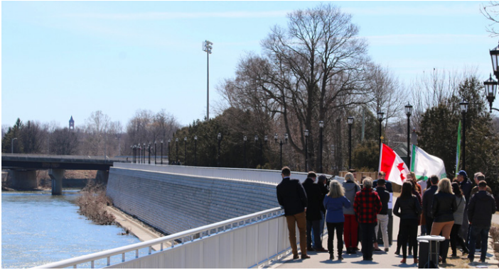
The federal funding announcement took place on a recently reconstructed section of the West London Dyke, north of the Queens Avenue bridge over the North Thames River.
