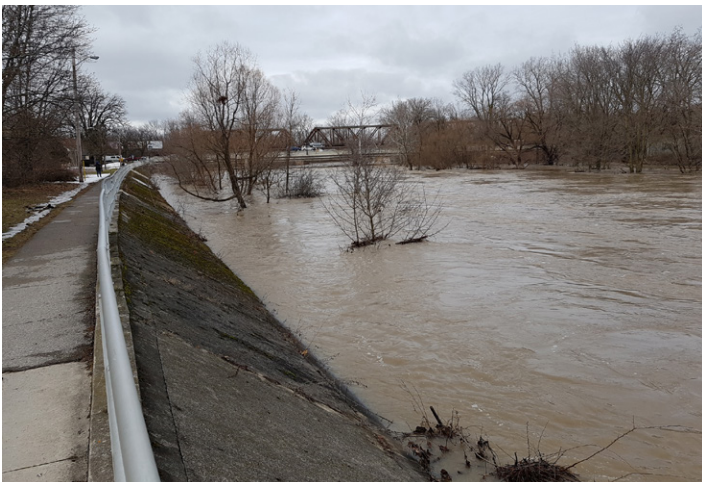
The project will include the reconstruction of approximately 1,600 m of the dyke, including this section near the Oxford Street West bridge, pictured during the February 2018 flood.
