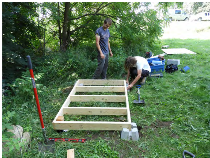
Installing a shed to house monitoring equipment next to Kintore Creek.
