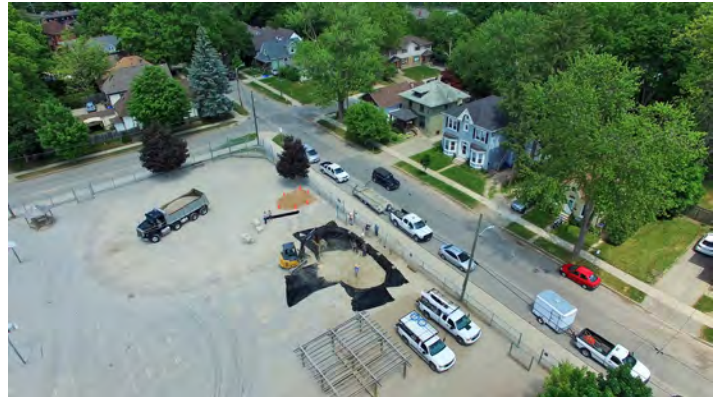
A rain garden was installed at Jeanne-Sauve French Immersion Public School.
