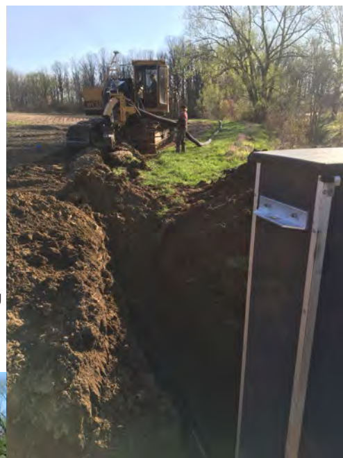
The control structure directs flows from the upland subsurface tile drainage system into perforated tile drains running along the stream edge for about 250 metres in both direction.
