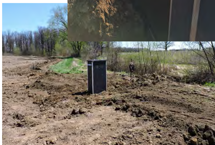
The control structure directs flows from the upland subsurface tile drainage system into perforated tile drains running along the stream edge for about 250 metres in both direction.
