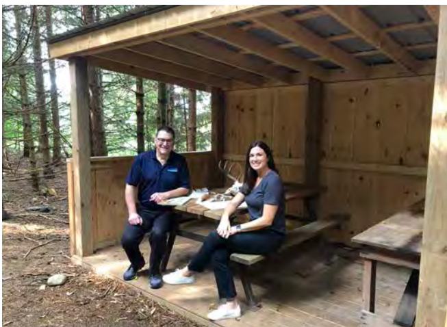
Local business owner Jenny Roth and UTRCA’s Vanni Azzano in the newly constructed shelter.
