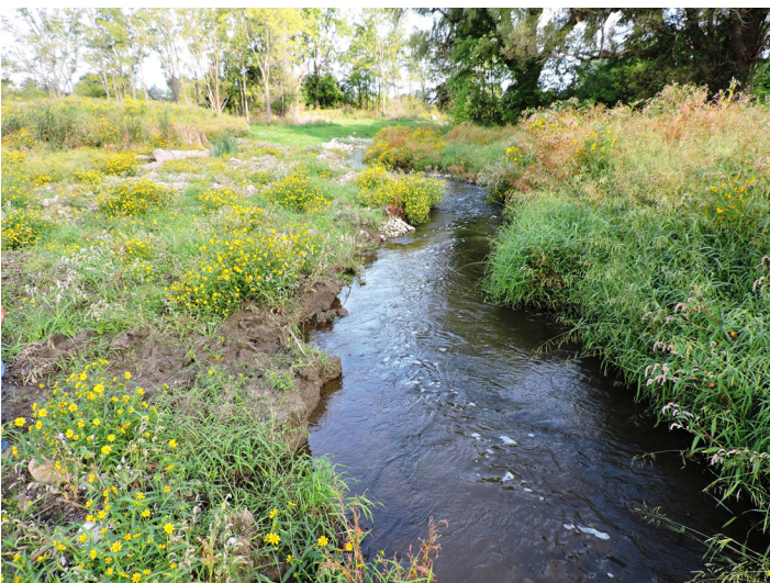
Looking downstream along the new constructed channel and stone riffle.
