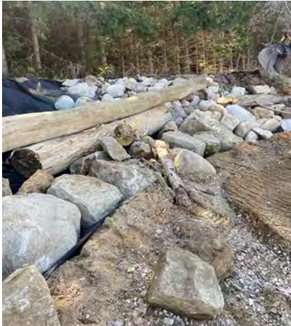
Along the asphalt pathway just east of Roth Park, large tree trunks or boles were built right into the bank revetment, in a visually appealing and environmentally friendly solution.
