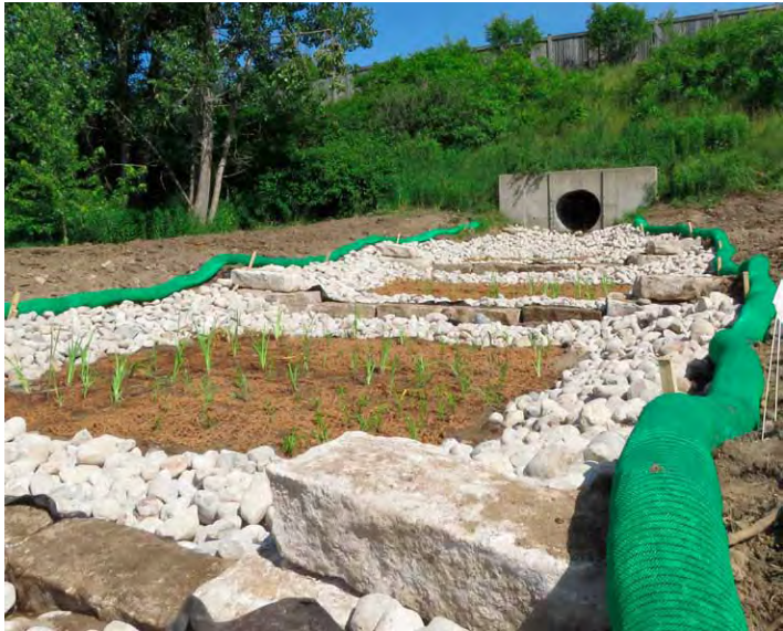
The Pittock biofilter has been planted with 300 native aquatic plants.
