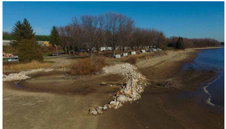
A drone view of the new rock shoal, which will be underwater during much of the year.
