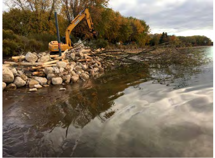
An 80 metre long shoal of rock and timber nears completion.
