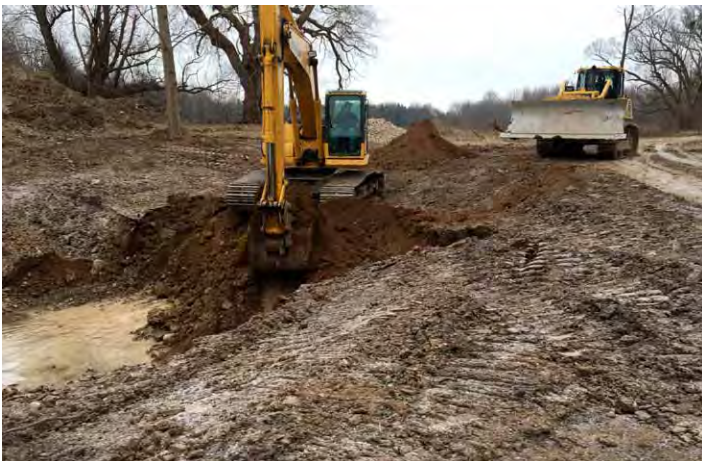
Digging a new channel from the creek towards the existing pond.
