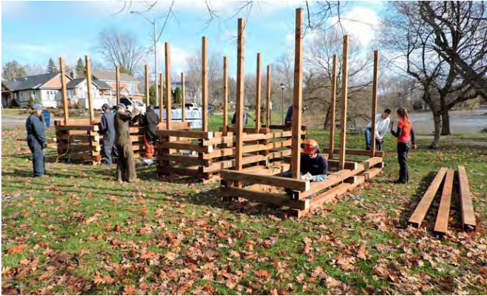
UTRCA staff enjoy a day of hard work and late season warm weather building 16' x 6' x 5' high timber cribs.
