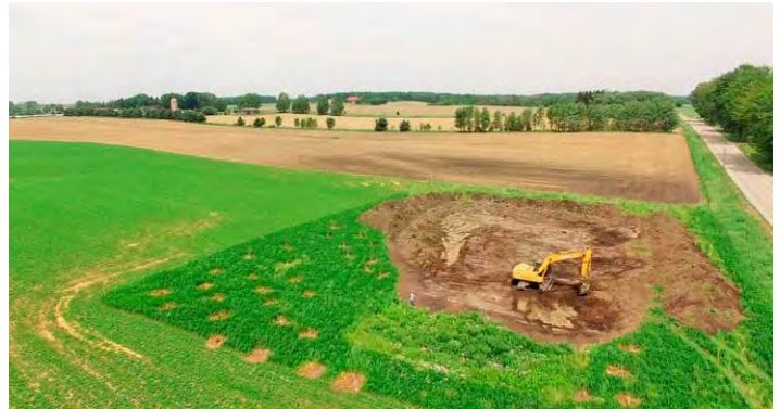
Aerial view of the wetland under construction.
