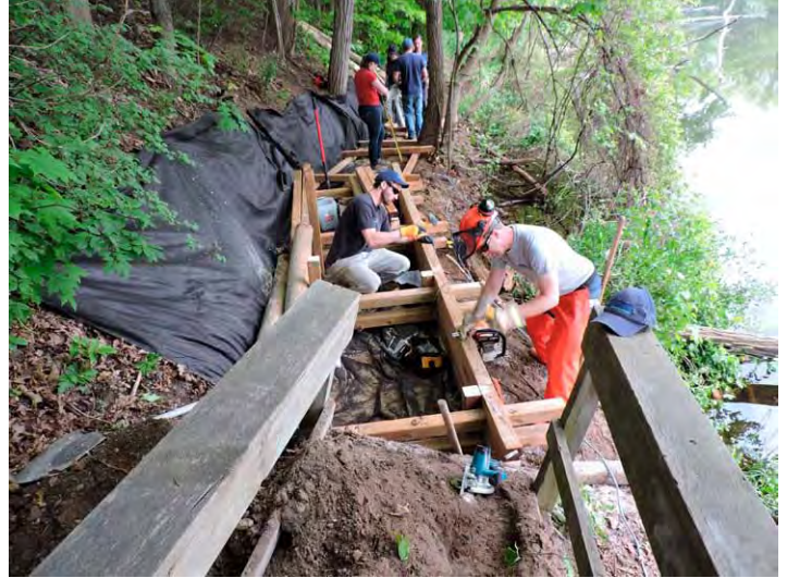
Building the timber cribs.
