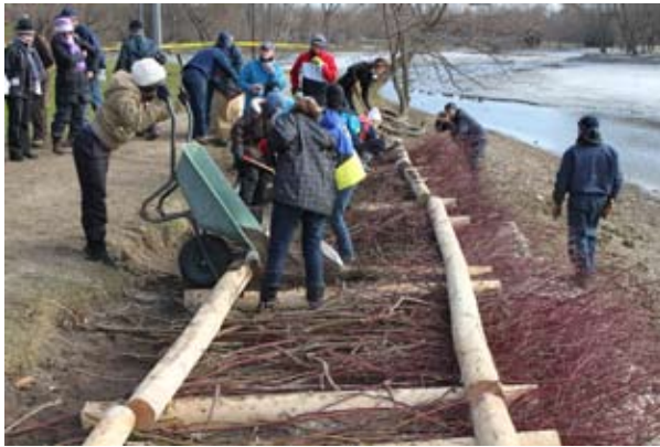
Students and UTRCA staff work on a bioengineering structure on Victoria Lake to protect the bank from erosion.
