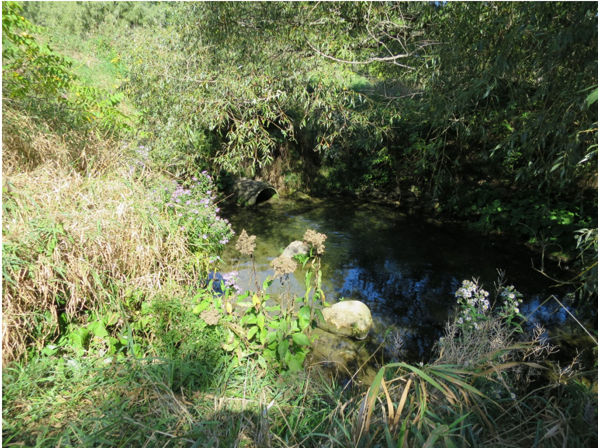
Photo 13. Youngsville Drain downstream of the dam
