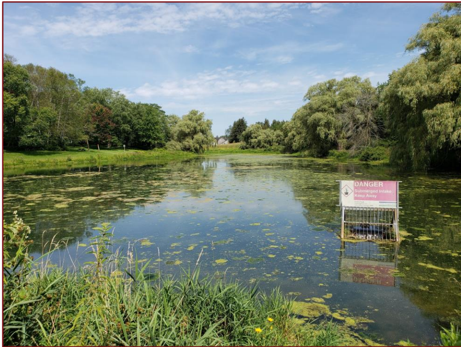
Image 9: Southwest Corner of Dam
