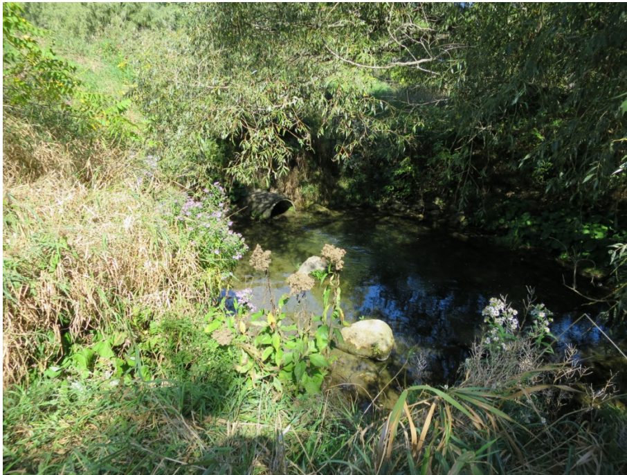
Photo 13. Youngsville Drain downstream of the dam
