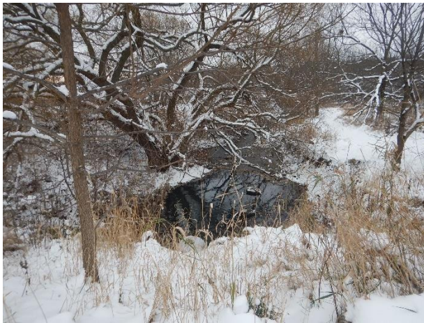
View downstream from dam outlet (2022).
