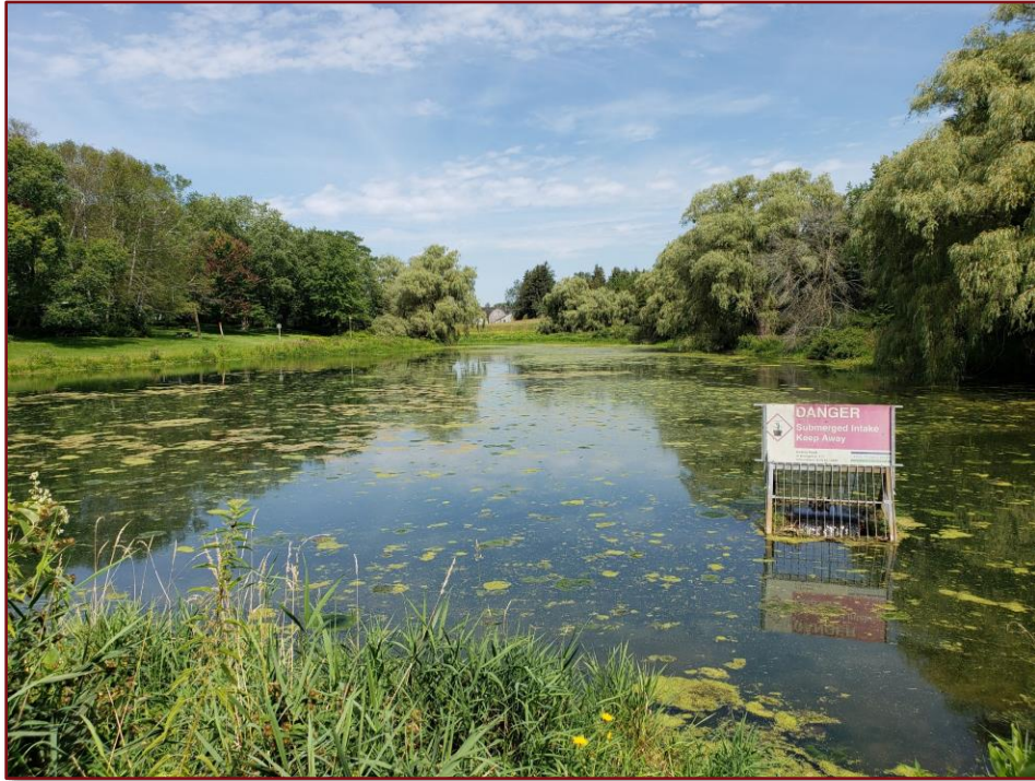
Image 9: Southwest Corner of Dam
