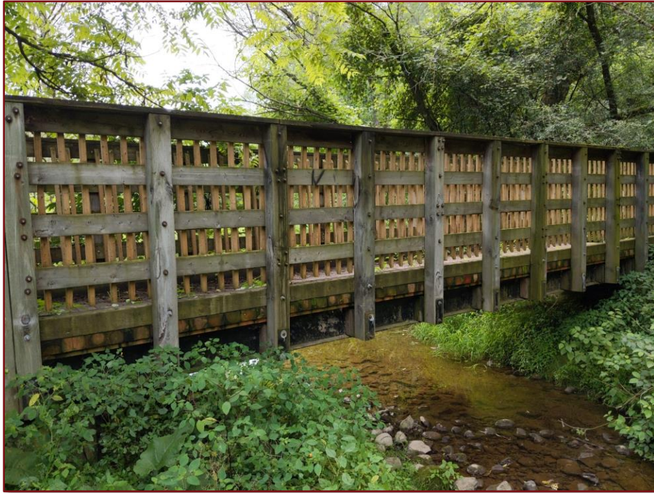
Image 13: Pond from Centre with View of Dam
