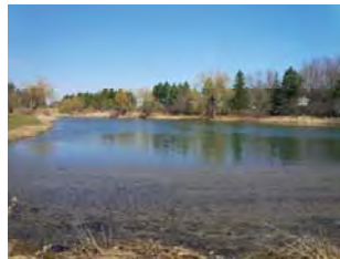
The dam contains water year round and includes approximately 3.4 m of head acting across the dam.
