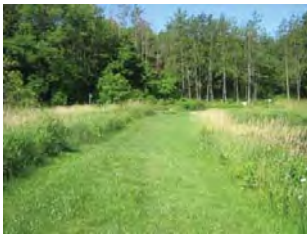
The Embro Dam is approximately 100 m in length, 4.5 m in height and includes 1.1 m of freeboard. The entire dam is founded on overburden as opposed to bedrock or engineered soil.
