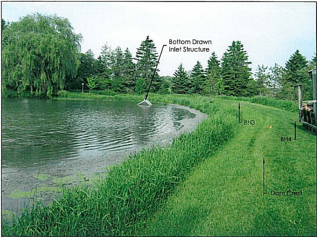
Photo 2: Looking east from west end of dam berm.
