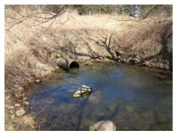
A 762 mm diameter (inner) concrete pipe conveys flow from the pond to a pool at the creek outlet.
