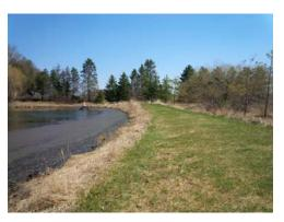
Low earth fill embankment, a grassed, emergency spillway is located at the east end of the embankment. This spillway has a clear width of about 4.0 m and the inlet invert is 0.6 m below the crest of the dam.
