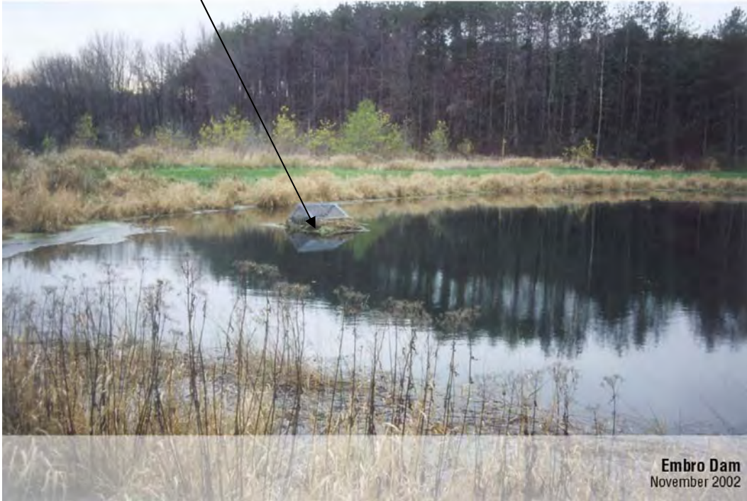
Photo 8 – Upstream Face of Dam
