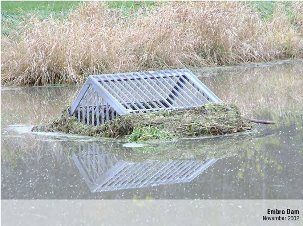
Photo 6 – Bottom Draw Inlet Structure
