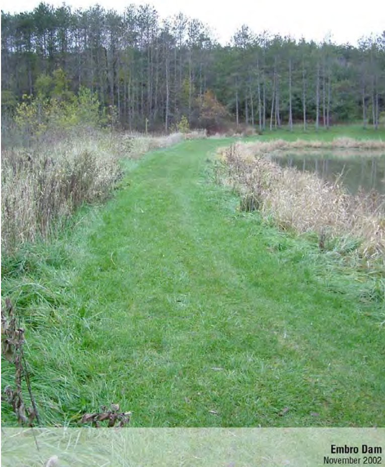
Photo 9 – View along Dam Crest
