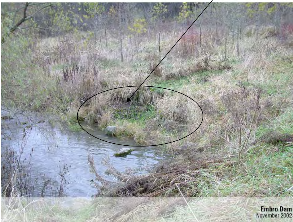
Photo 11 – Erosion along Right Downstream Channel
