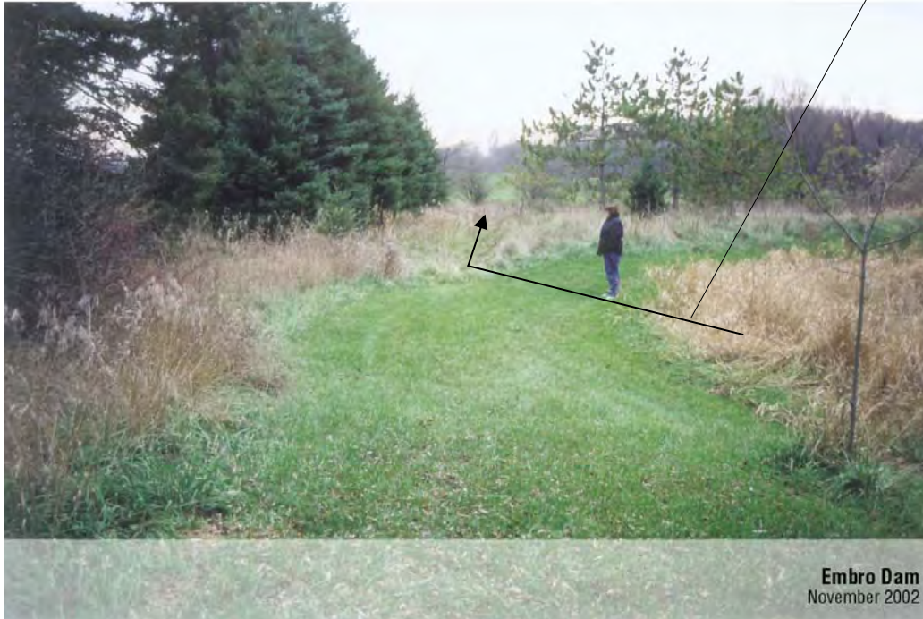
Photo 3 – Emergency Spillway Entrance
