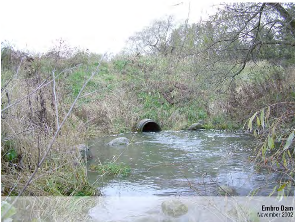
Photo 2 – Downstream View of Embankment at Pipe Outlet
