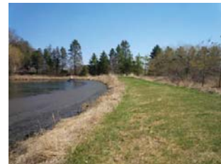
Low earth fill embankment, a grassed, emergency spillway is located at the east end of the embankment. This spillway has a clear width of about 4.0 m and the inlet invert is 0.6 m below the crest of the dam.
