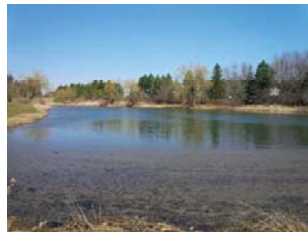
The dam contains water year round and includes approximately 3.4 m of head acting across the dam.
