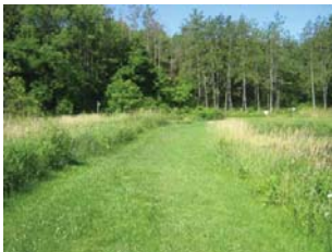
The Embro Dam is approximately 100 m in length, 4.5 m in height and includes 1.1 m of freeboard. The entire dam is founded on overburden as opposed to bedrock or engineered soil.
