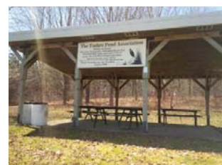
The Embro Dam is located within the Embro Conservation Area, with recent restoration and improvement works undertaken by the Embro Pond Association.
