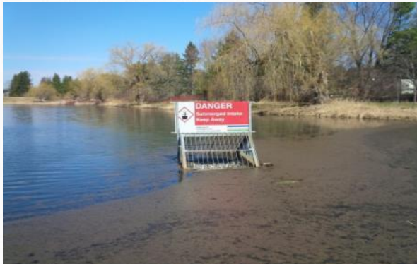
The outlet of the dam includes a concrete bottom draw inlet structure covered with grated trashrack.
