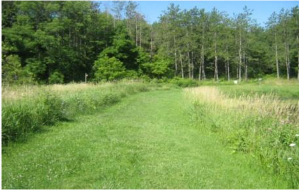
The Embro Dam is approximately 100 m in length, 4.5 m in height and includes 1.1 m of freeboard. The entire dam is founded on overburden as opposed to bedrock or engineered soil.
