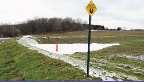
This broad- based berm was constructed in 2015. Signage is useful to notify custom farm operators of the location of erosion control structures.
