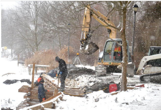
Staff and contractors with the Upper Thames River Conservation Authority worked to complete construction on a number of shoreline improvements along Lake Victoria's north shore in Stratford Friday morning. Improvements include making a 60-metre stretch of the city's north-shore pathway more accessible, constructing wooden cribbing and reinforcing the shoreline with rocks to prevent further erosion, and building a kayak and canoe launch closer to the water to make it easier to get in and out from shore. Galen Simmons/The Beacon Herald/Postmedia Network
