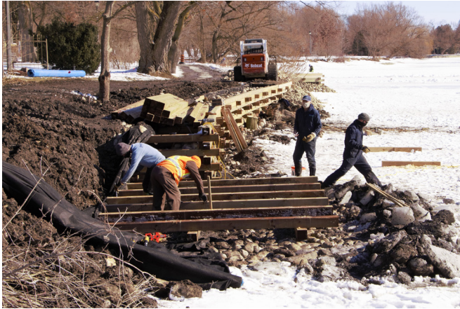
The accessible canoe/kayak launch and erosion control are constructed of a timber cribwall with underwater rock shoals.
