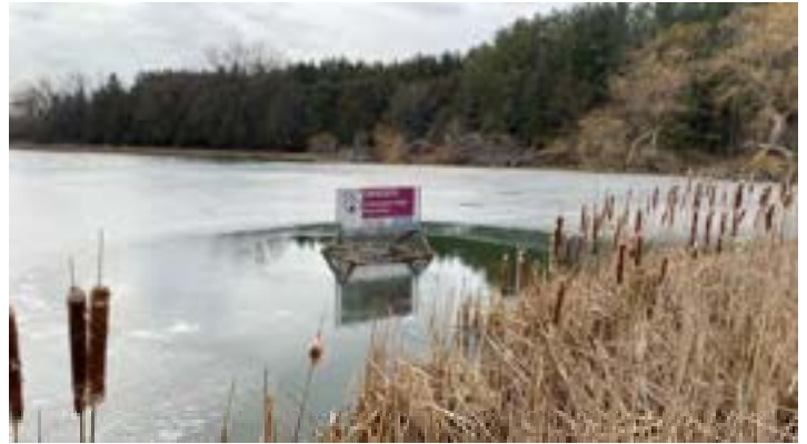
Photo 2: Reservoir Drop Inlet Structure.
