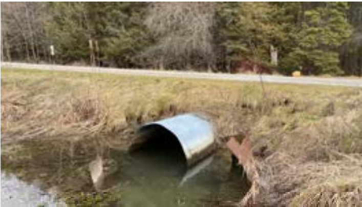
Photo 21: Perth Road 163a culvert.
