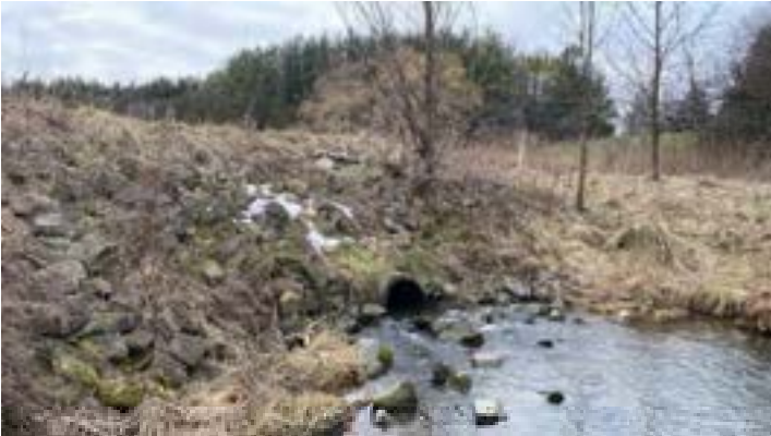
Photo 3: Reservoir outlet structure.
