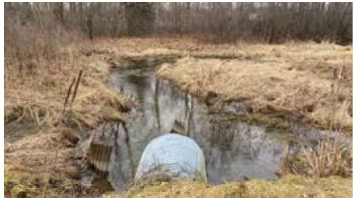
Photo 6: Reach 1 looking upstream from Perth Road 163a culvert.
