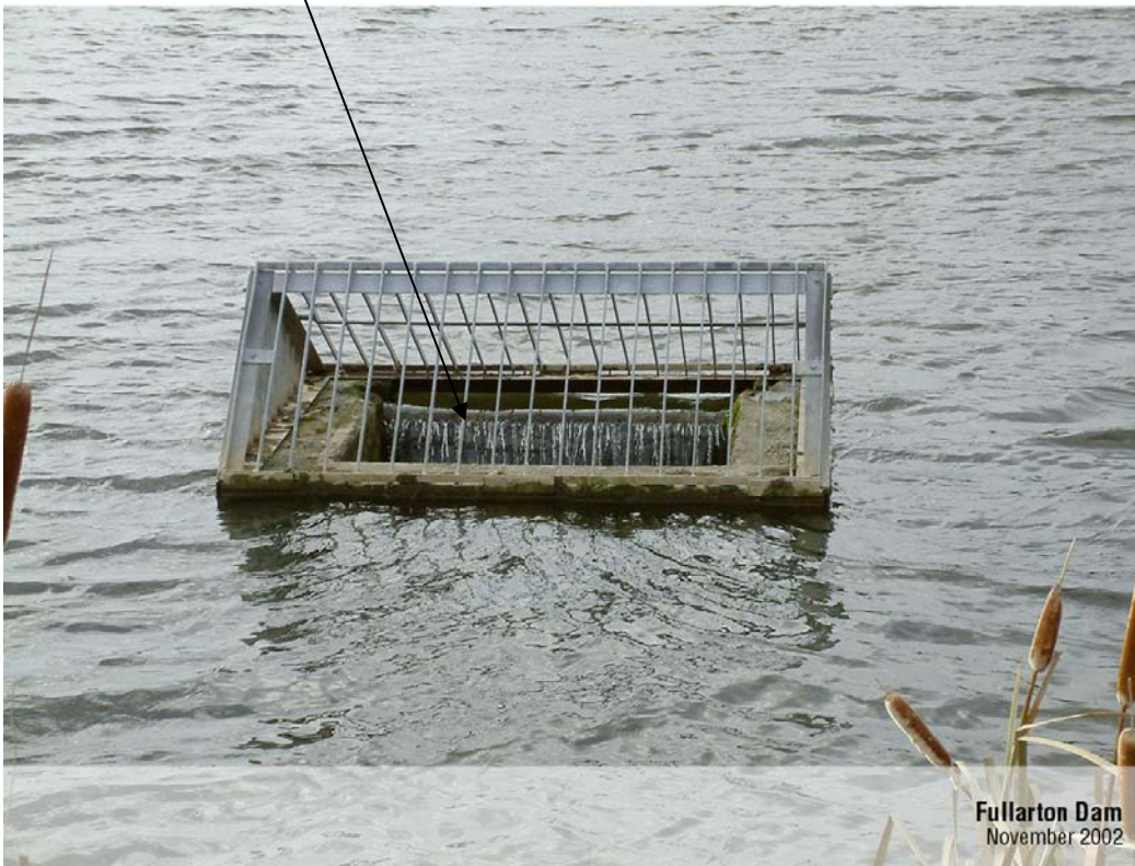
Photo 12 – Drop Inlet Structure
