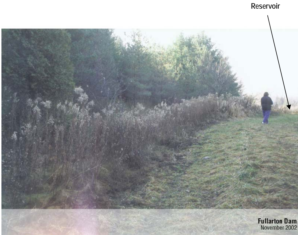
Photo 7 – Upper Reach of Emergency Spillway Channel
