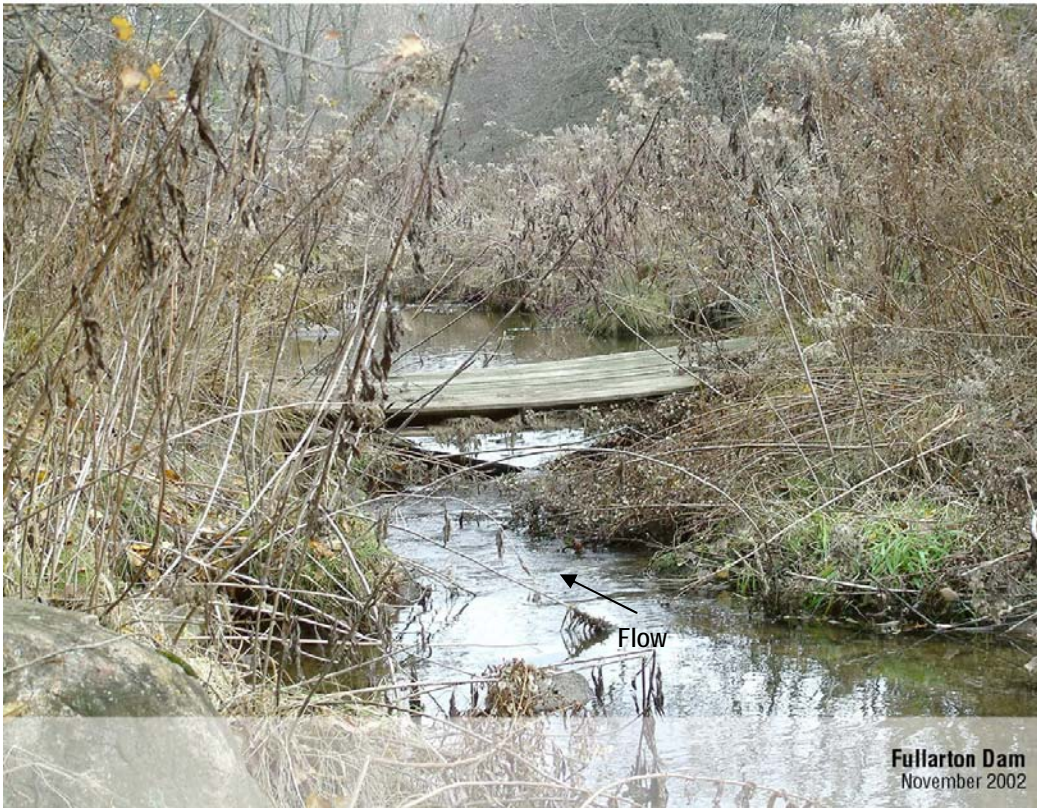
Photo 8 – Wood Footbridge Across Downstream Channel
