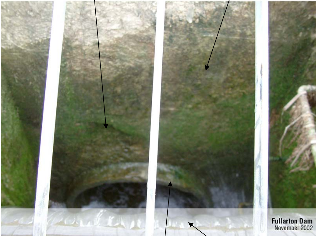
Photo 13 – Inside of Drop Inlet Structure
