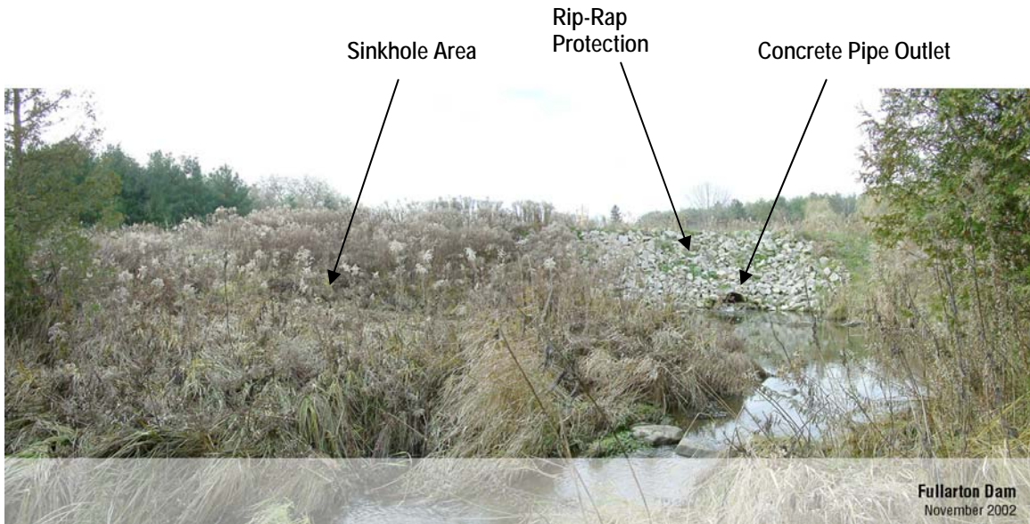
Photo 4 – Downstream View of Dam
