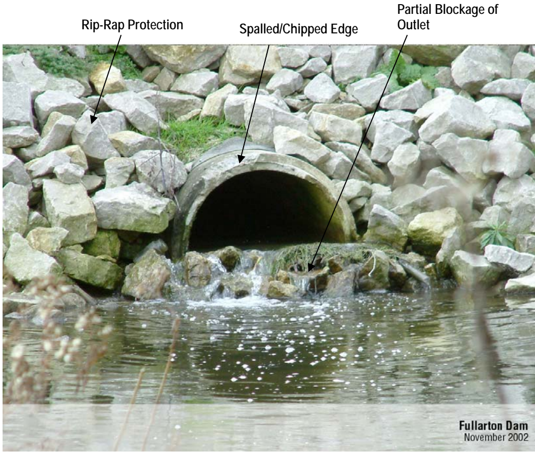
Photo 11 – Close-Up of Outlet Pipe
