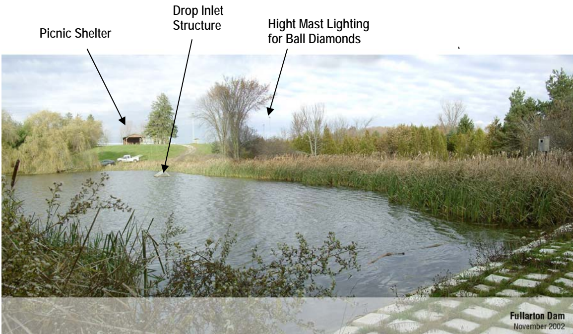
Photo 9 – Upstream Face of Dam
