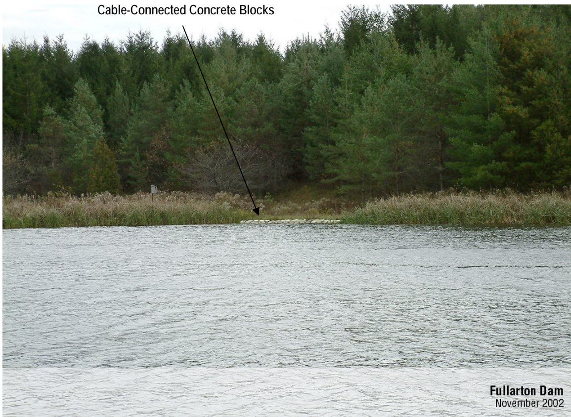
Photo 5 – View of Emergency Spillway Entrance
