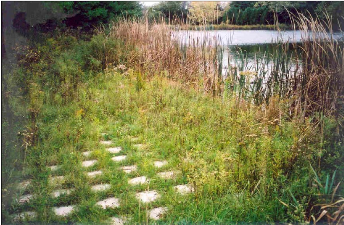
Photo 2: Overflow spillway located southeast of the dam.
