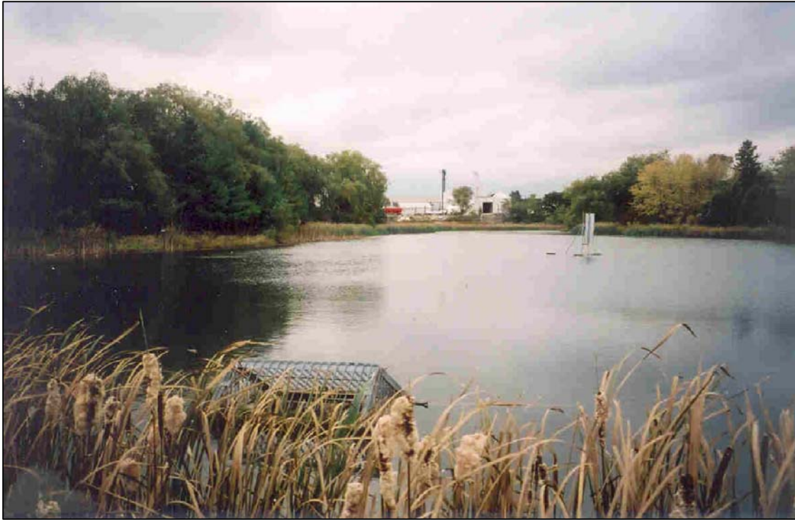
Photo 3: Looking south towards the pond and the drop inlet structure.
