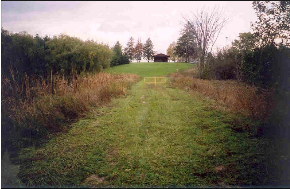
Photo 1: Looking west along the top of the dam.
