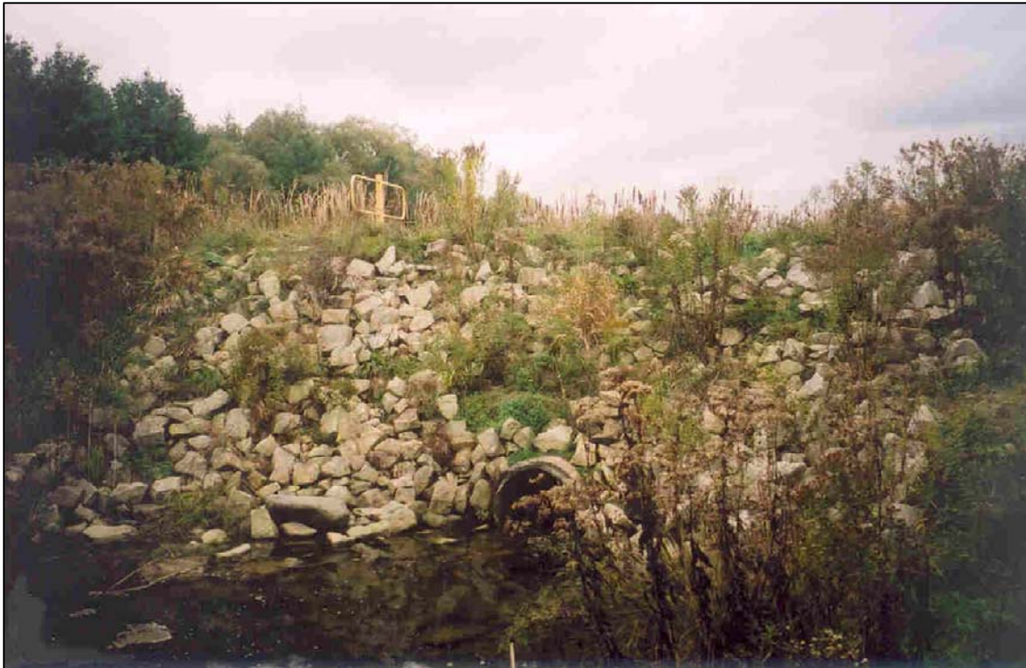
Photo 4: Outlet pipe on the north side of the dam.
