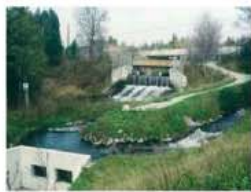
MEANDERING FISHWAY AROUND DAM
