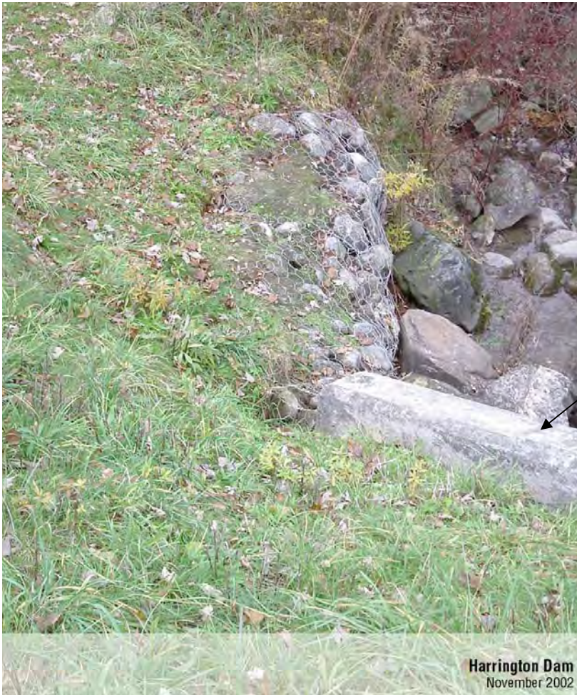
Photo 8 – Gabion Baskets, Left Downstream Side of Spillway
