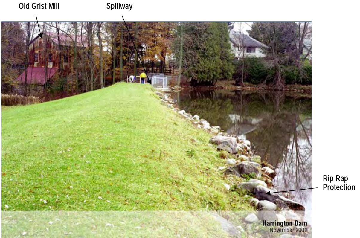
Photo 11 – Upstream Slope and Crest of Left Embankment
