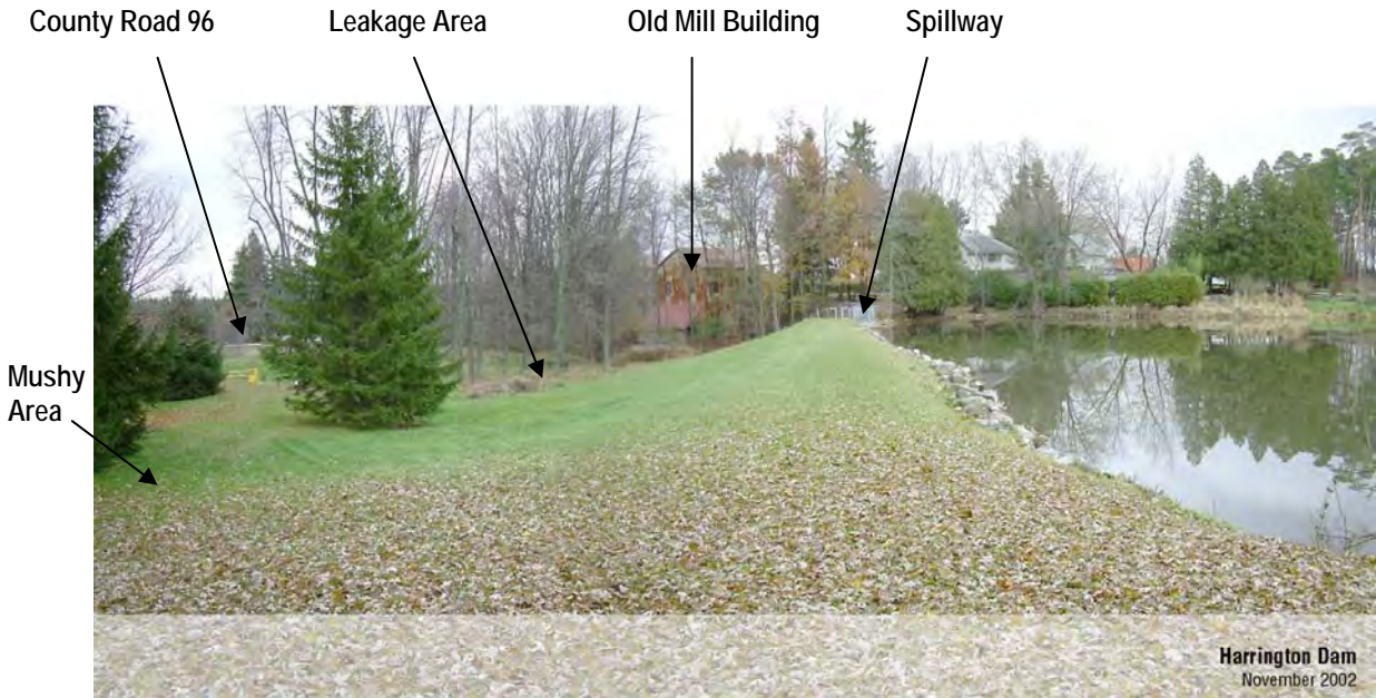
Photo 1 – View of Dam from Right Bank
