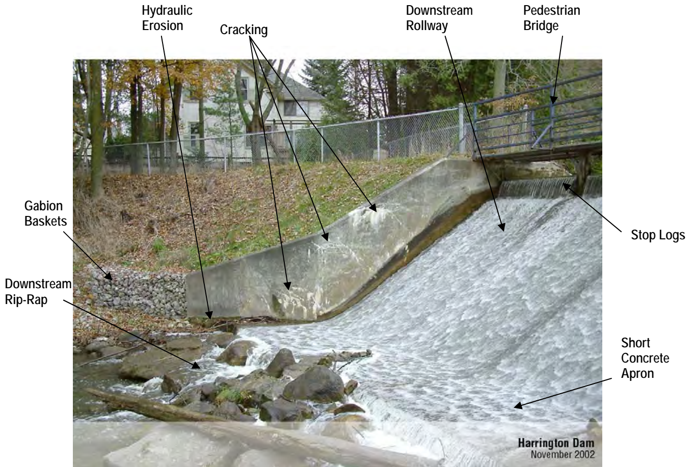
Photo 2 – Downstream View of Right Embankment
