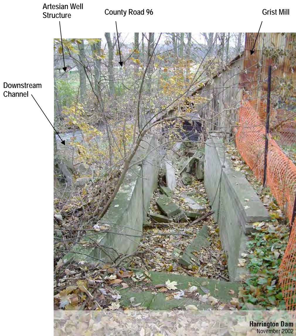
Photo 19 – Concrete Flume Leading to Grist Mill
