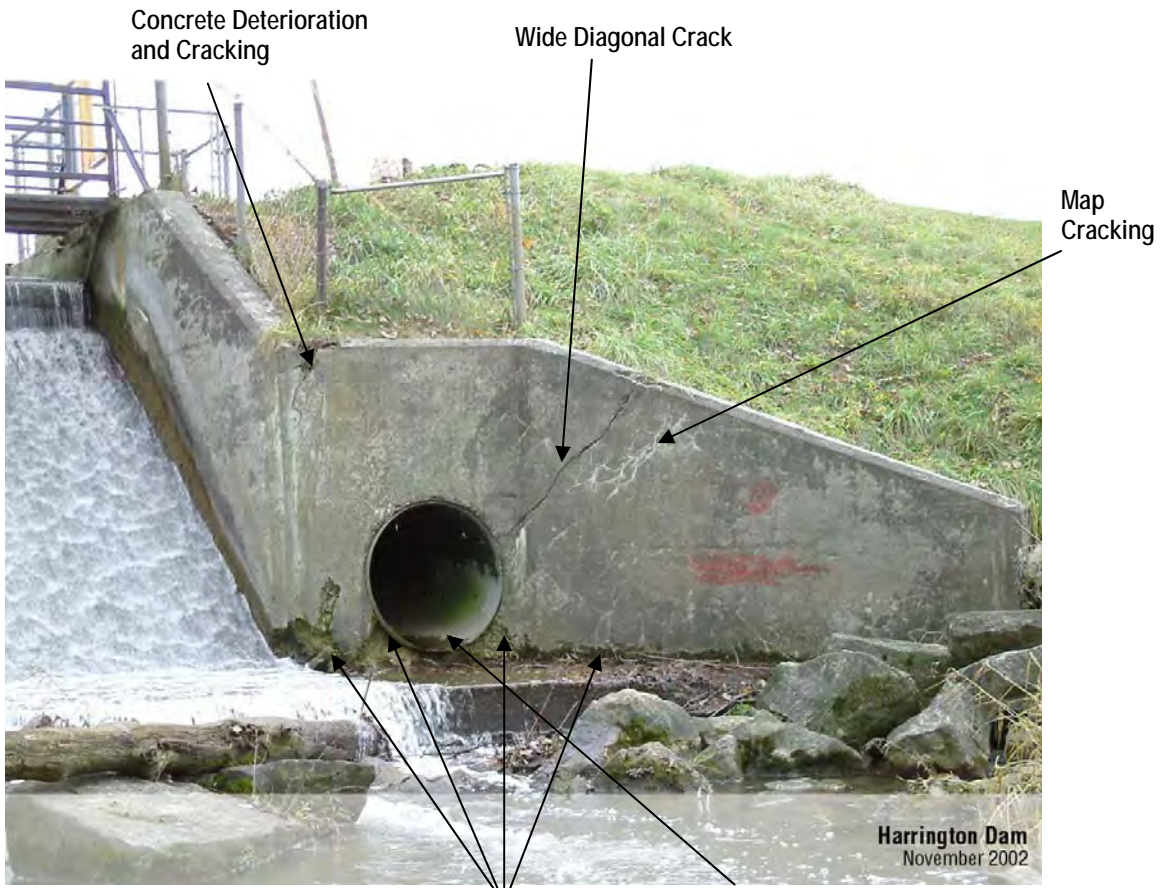
Photo 17 – Left Downstream Wingwall
