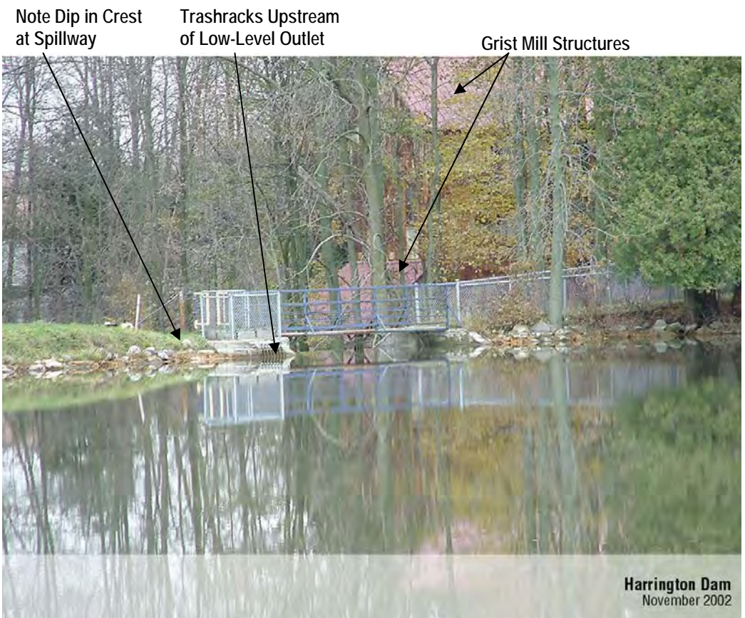
Photo 13 – Upstream View of Spillway
