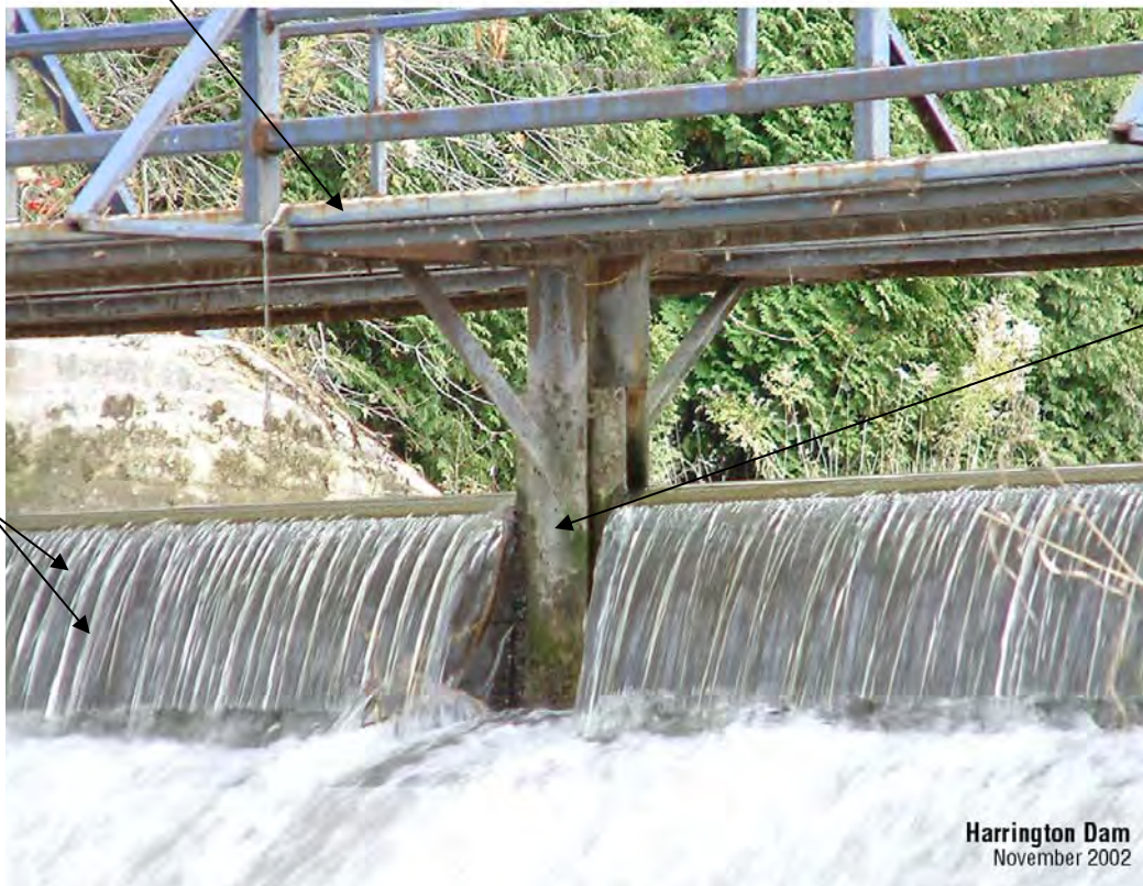
Photo 18 – Intermediate Piers of Spillway
