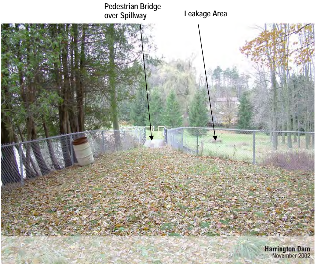
Photo 14 – Crest of Right Embankment
