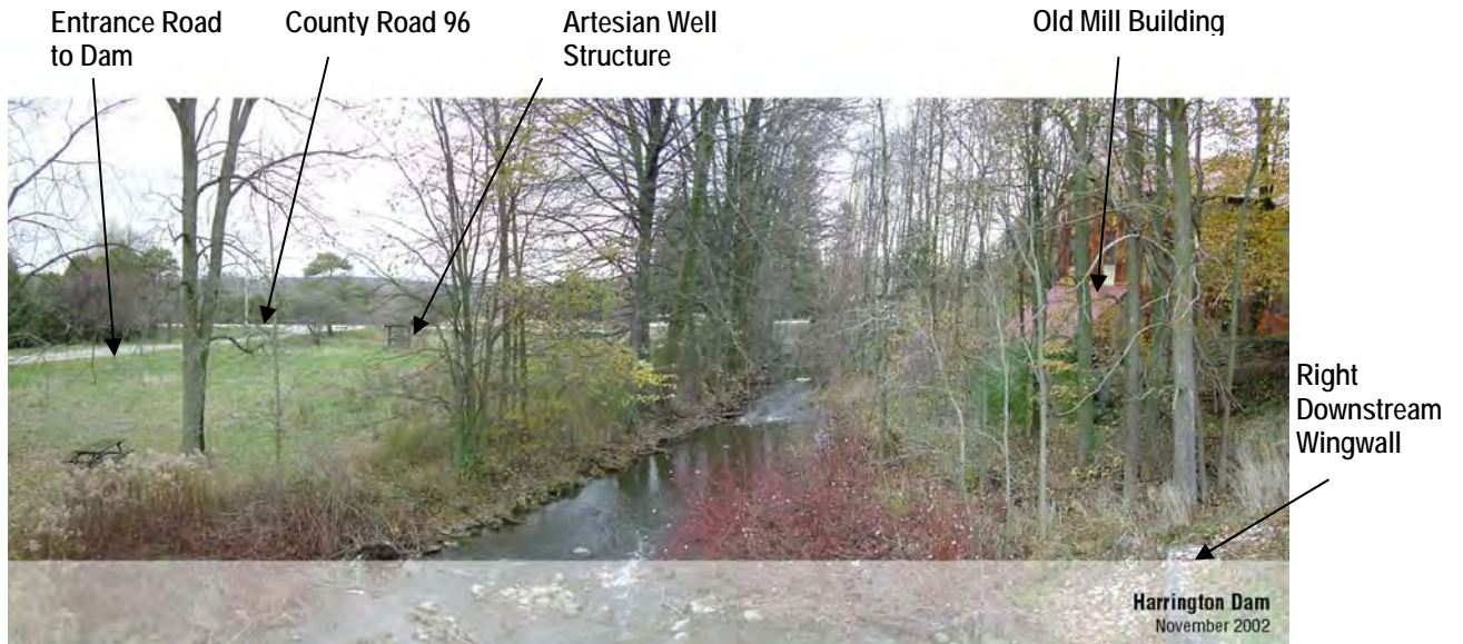
Photo 5 – Area Downstream of Dam
