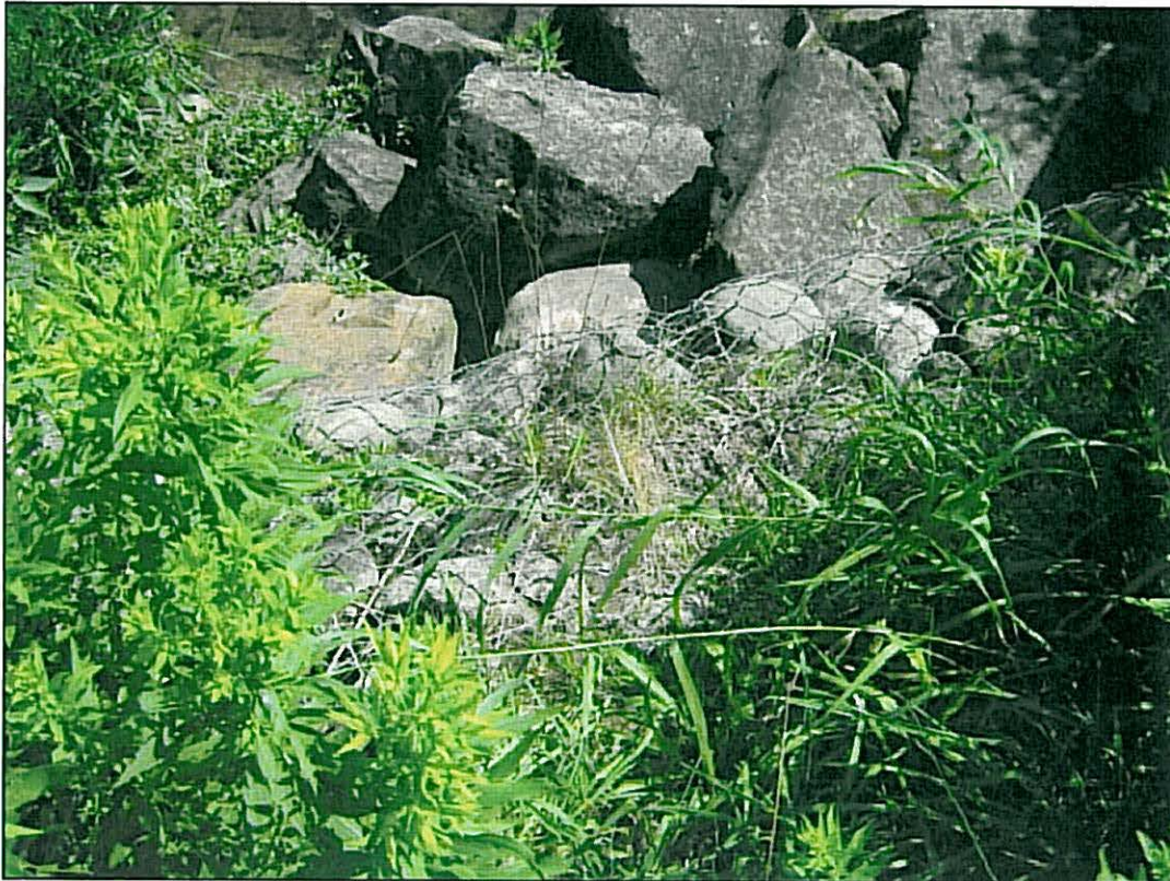
Photo 6: Rip rap lining the creek channel immediately downstream of the dam.
