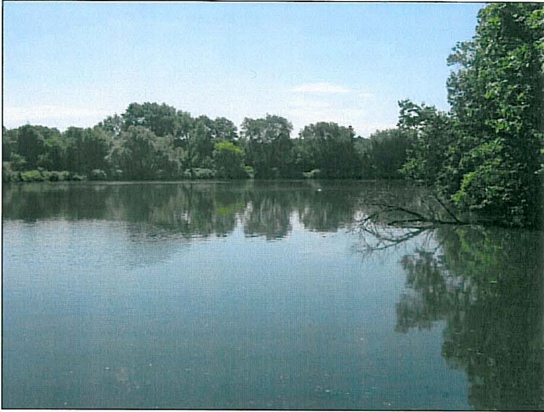
Photo 3: Looking south over the dam reservoir.
