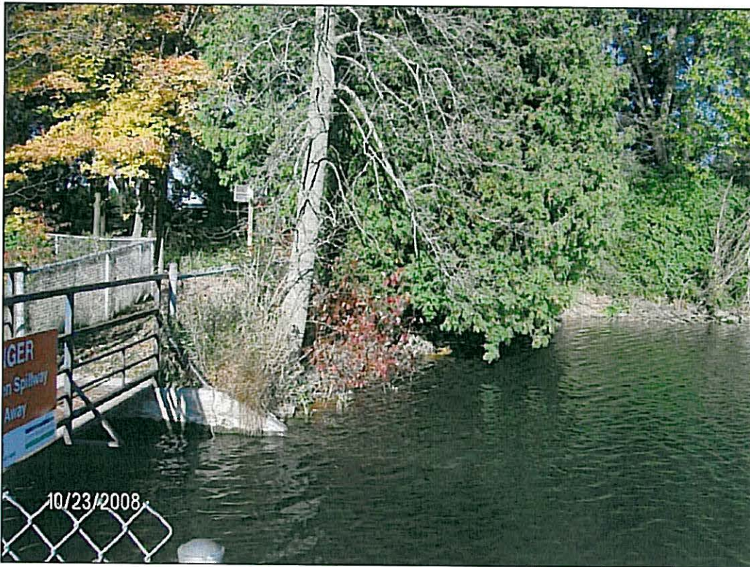
Photo 10: Trees at east embankment.
