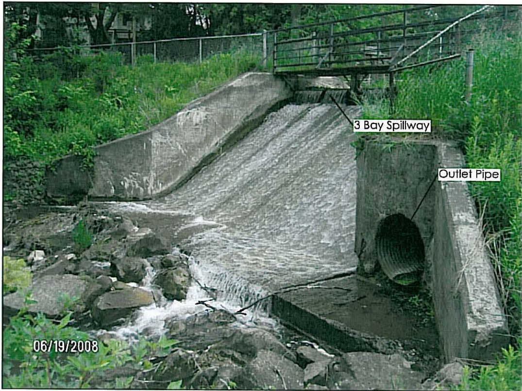
Photo 8: Looking southeast at the dam structure.
