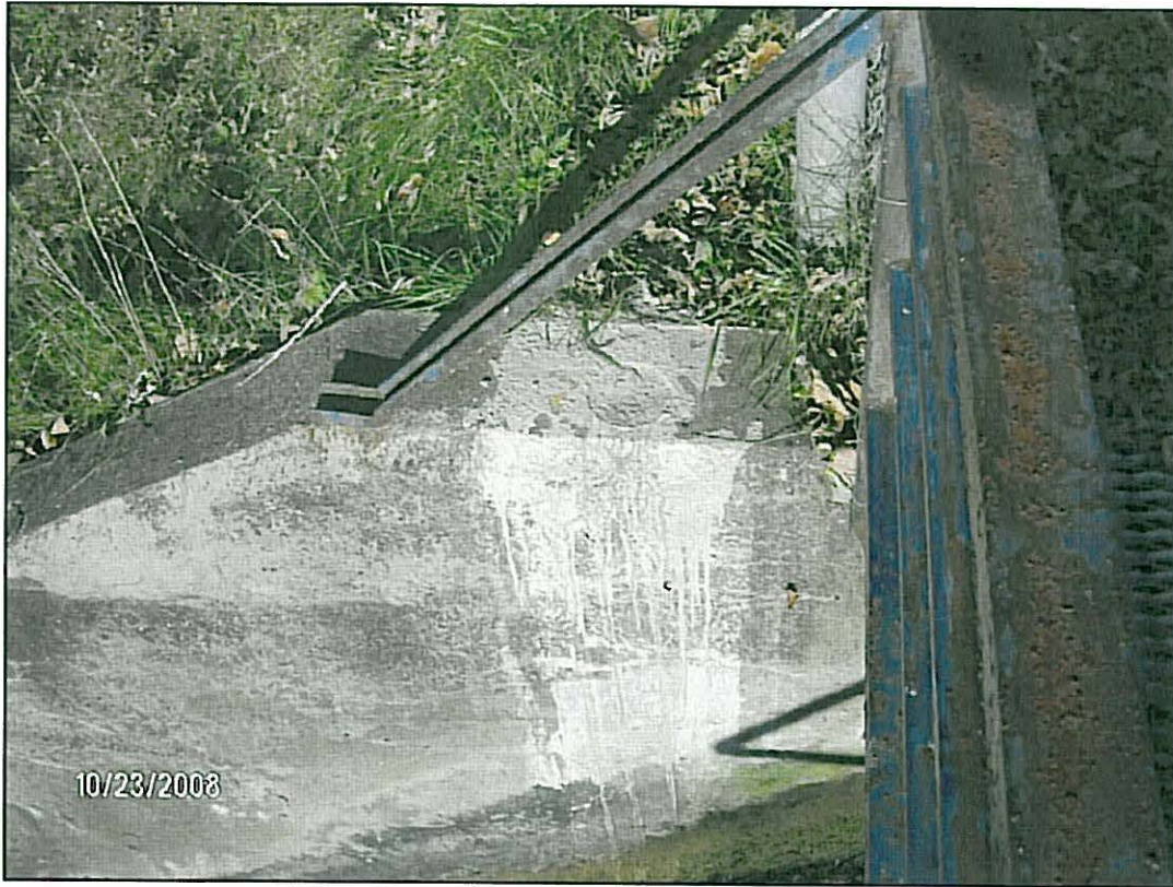
Photo 13: Concrete corehole at east wall.
