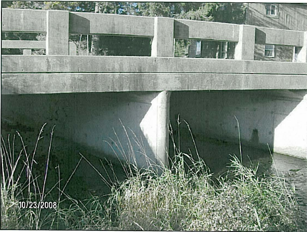
Photo 17: Twin box culvert at Road 28.
