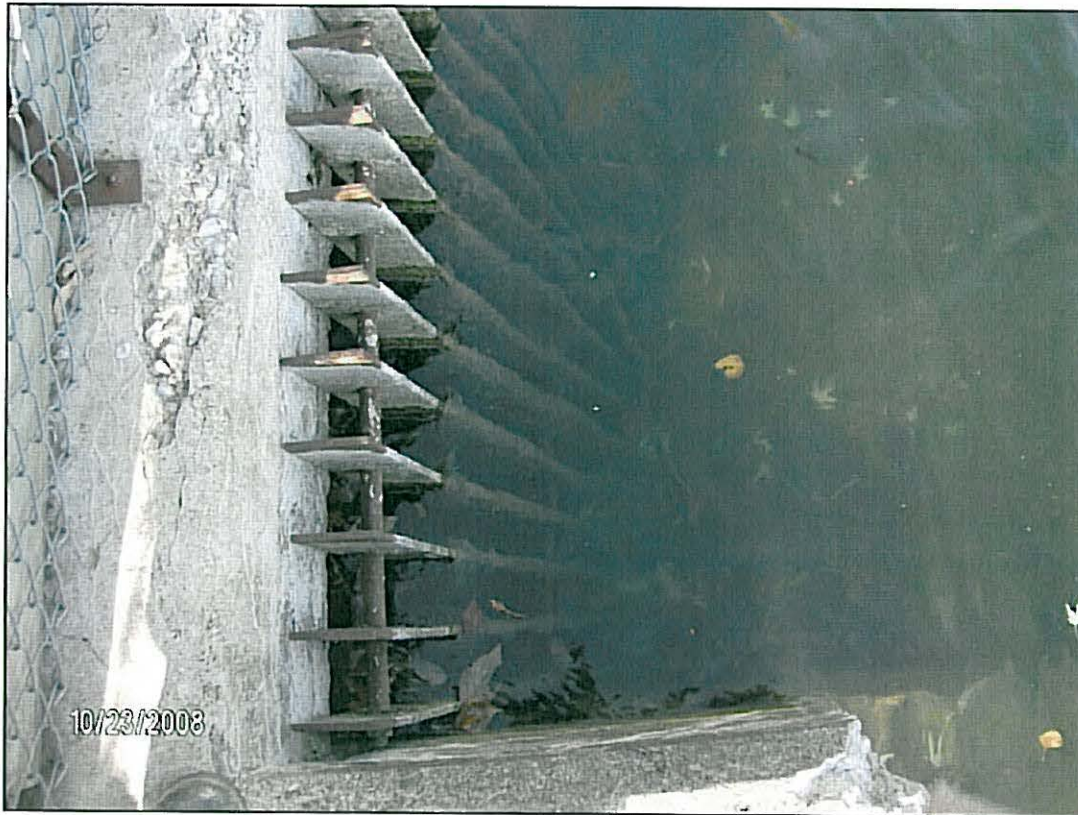
Photo 14: Culvert inlet at west wall.
