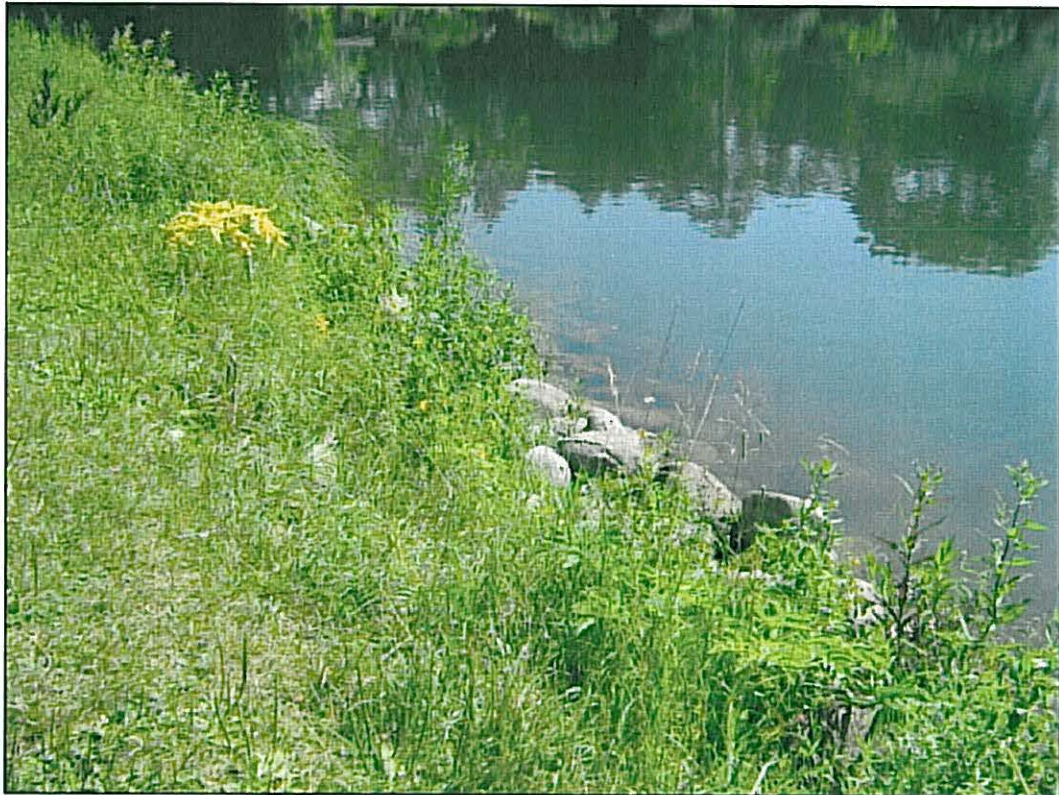
Photo 4: Showing the rip rap located on the south (pond) side of the embankment.
