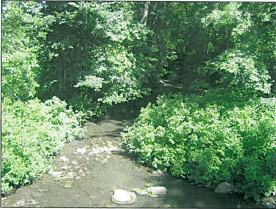
Photo 7: Looking north towards the stream downstream of the dam.
