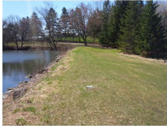
The earthen embankments of the dam are founded on soil overburden, rather than bedrock or engineered soil.
