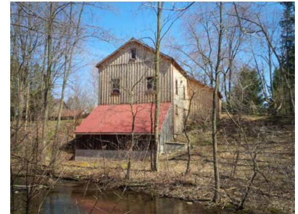
The Harrington Dam is located within the Harrington Conservation Area; the adjacent mill building has recently been restored by the Harrington Community Club.
