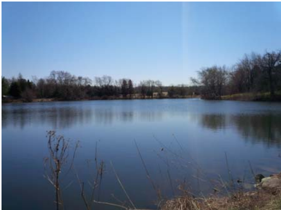
The dam contains water year round and includes approximately 3.3 m of head acting across the dam.
