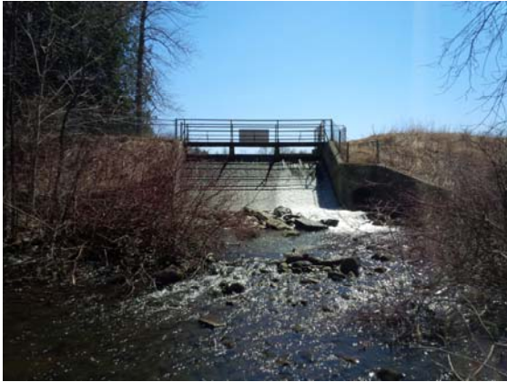
The Harrington Dam is approximately 90m to 95m long, with two earthen embankments flanking a concrete spillway.
