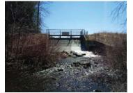
The Harrington Dam is approximately 90m to 95m long, with two earthen embankments flanking a concrete spillway.
