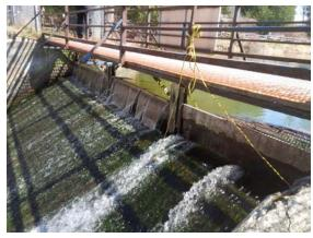
The dam spillway is considered to have an inadequate capacity for safety and stability purposes; the water level in the reservoir can be adjusted by adding stop logs to the spillway.
