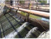
The dam spillway is considered to have an inadequate capacity for safety and stability purposes; the water level in the reservoir can be adjusted by adding stop logs to the spillway.
