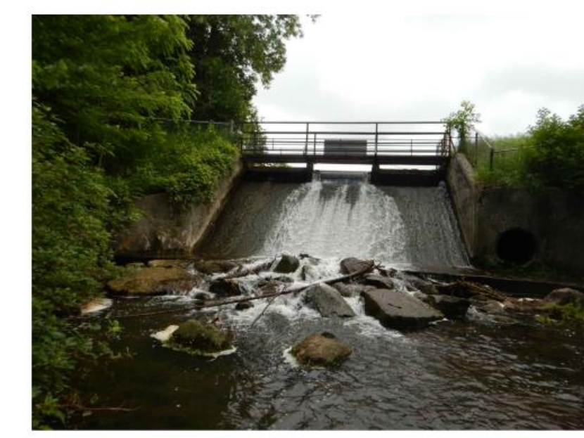
EXISTING HARRINGTON DAM
