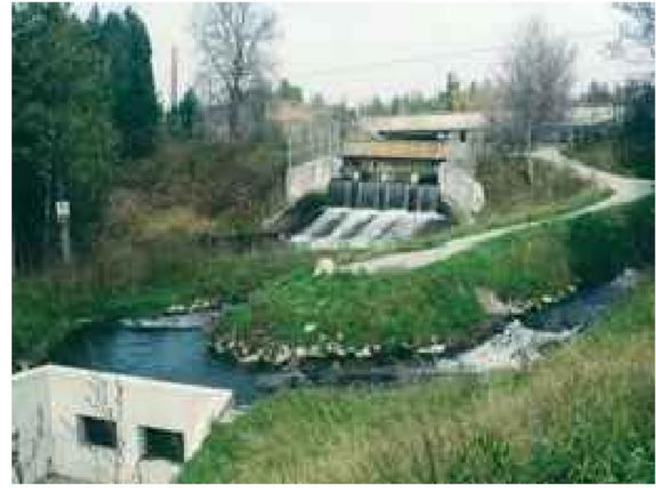
MEANDERING FISHWAY AROUND DAM
