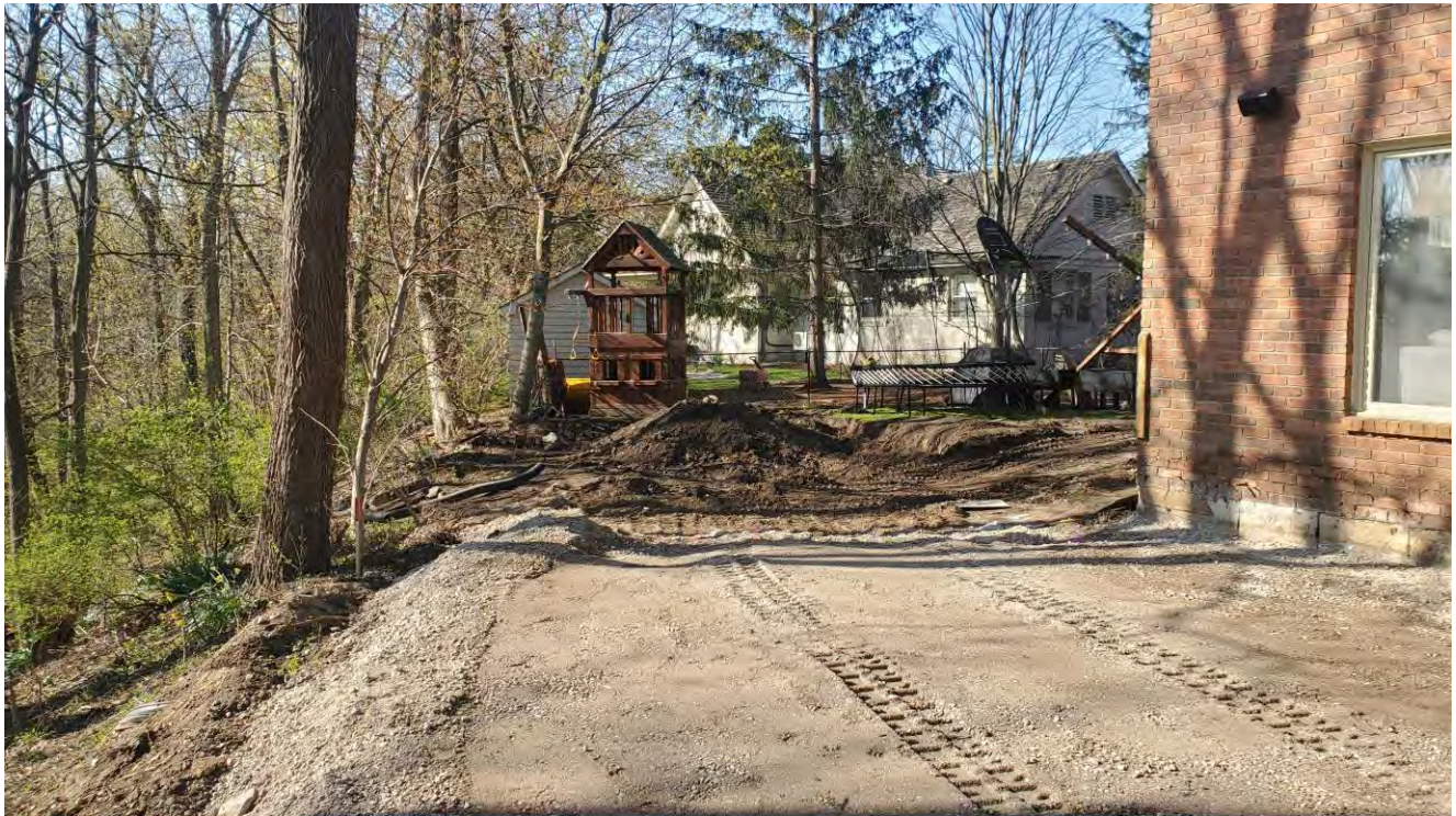
Photo 1 – Top of Existing Slope Near Proposed Cabana Location
