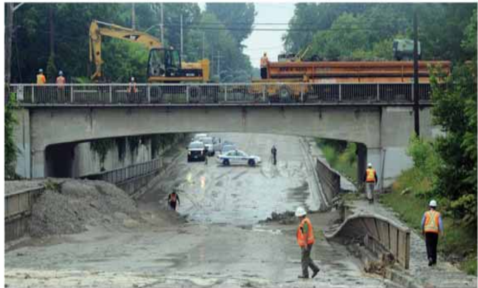
The Dixie Road underpass in Mississauga, Ontario, was one of many infrastructure assets damaged following the July 8, 2013 storm event. (Source: Fred Look, Mississauga News)
