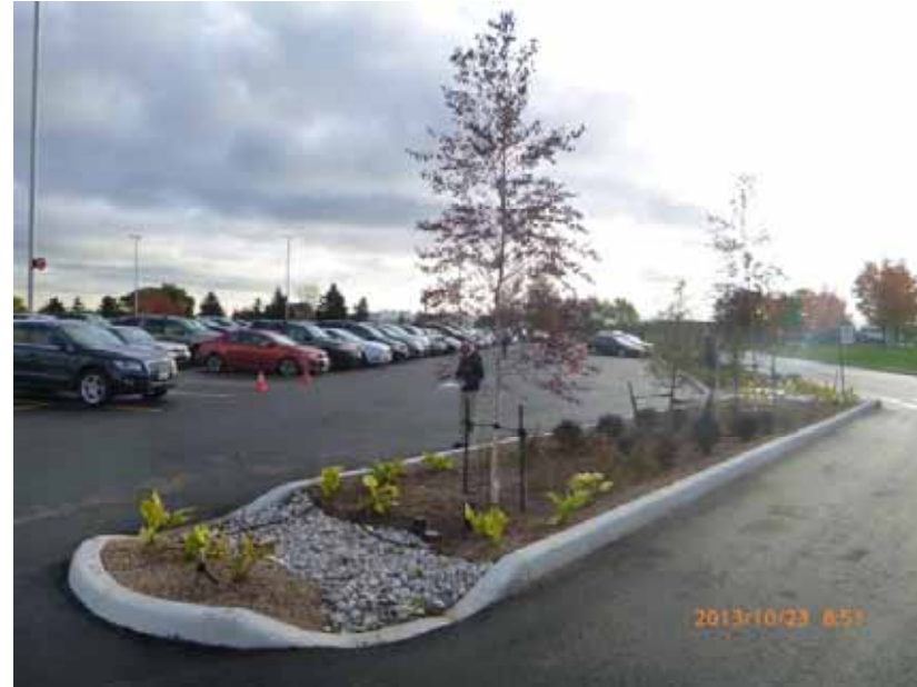
Fine grading of bioretention areas after planting to stop short circuiting
