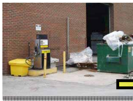
Fuel station spill pad
