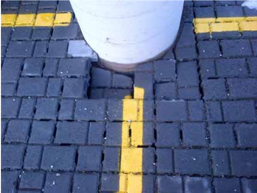
Compaction around light standards
