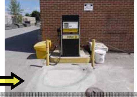
Fuel station spill pad
