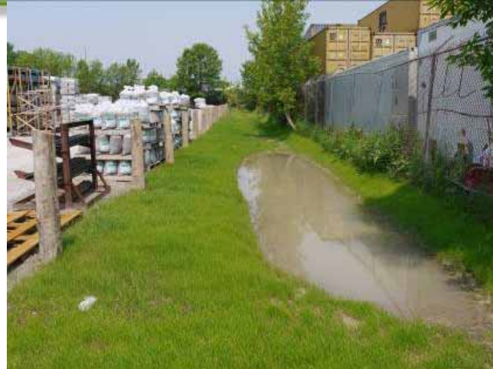
After Construction – after rain event
