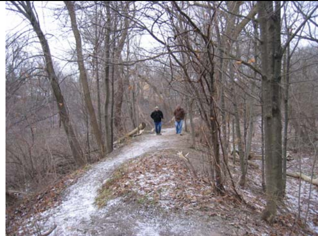
A mixture of immature Manitoba and Norway Maples growing on the Nelson-Clarence Dyke. Selective maintenance in 3-5 years will avoid more extensive maintenance or repairs in future.
