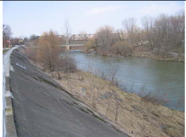
Regenerating vegetation in deposition zone south of Blackfriar Bridge. Monitoring should ensure that invasive species do not become established in gaps between concrete pads.
