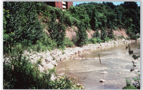
Figure 127- Protection Works for Confined System (example)
