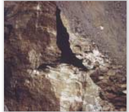
Figure 60 - Piping Hole
