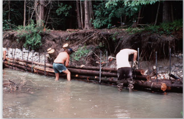
Figure 133 -Installation of Log Crib
