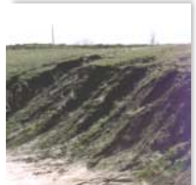
Figure 5 - Gully Erosion of Slope
