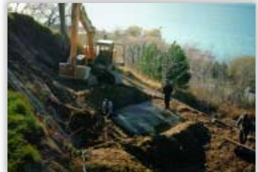
Figure 85 - Installation of Geomattng
