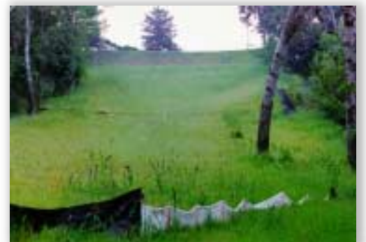
Figure 87 - Repaired Slope, Filled Slope Designed by Geotechnical Engineer
