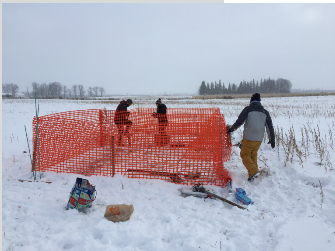
Building the snow fence (photo credit: Janina Plach)
