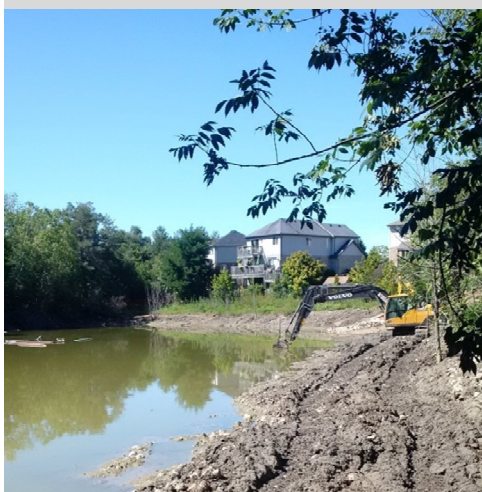
Maintenance of a Stormwater Management facility (photo credit: City of London)
